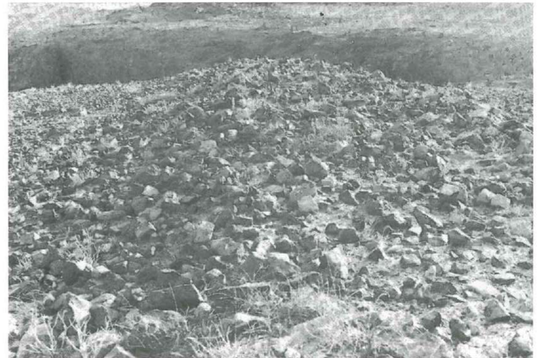
b. part of the city wall in the third sector, looking south-west (invent. no. MAIRAY-840122, A. de Maigret).
