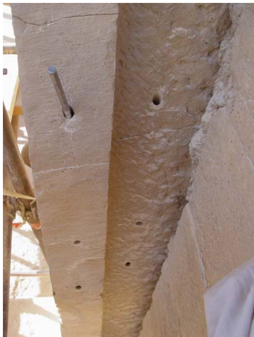
Fig. 30 Stainless steel bars were used to restore the two monolithic door jambs of the temple main entrance
