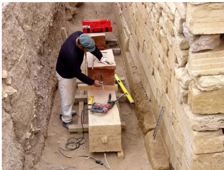
Fig. 28 Preliminary work for pinning the broken section of the monoliths
