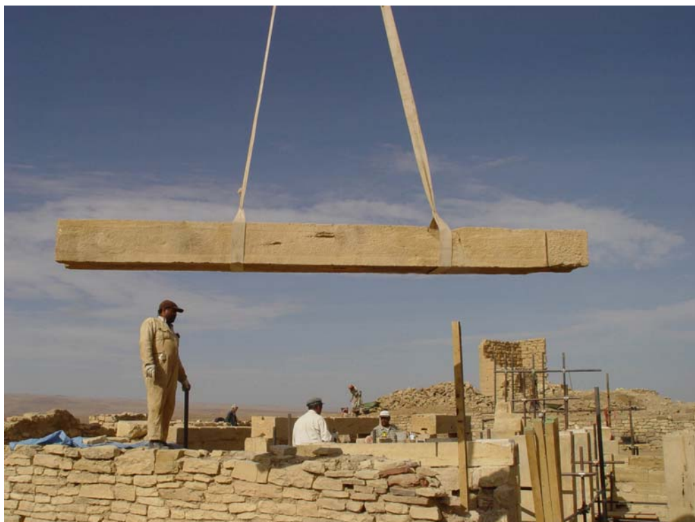
Fig. 31 One of the broader girders being reassembled in its original position
