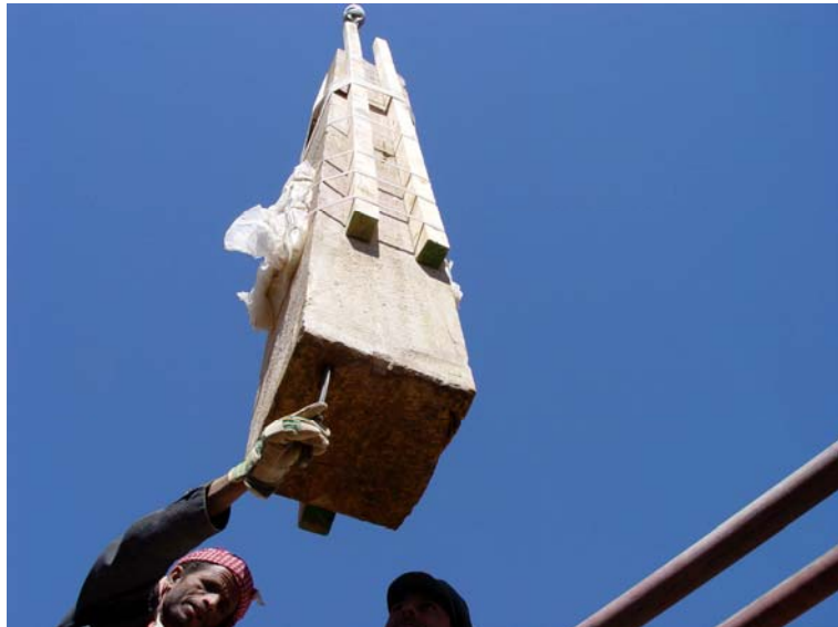
Fig. 27 The disassembly of one of the 12 pillars
