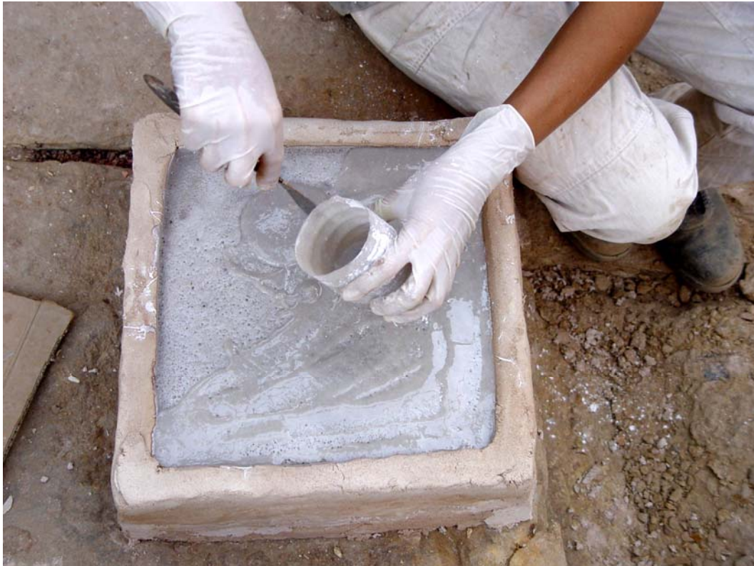
Fig. 29 Epoxy resins reinforced with quartzite were to construct new level plinths for the pillars
