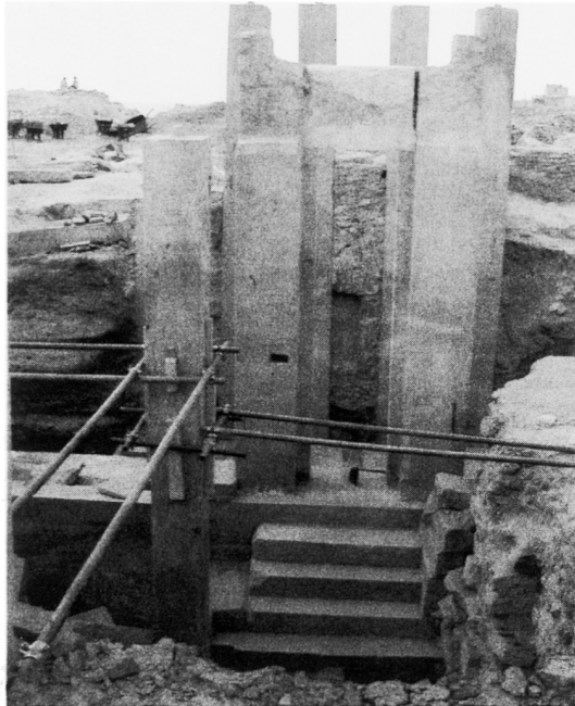
Photo G - Barāqish, Temple B. The staircase M105 leading down to the floor of the hypostyle hall.
