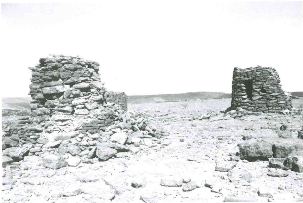
a. Necropolis MKDi. In this view of two tombs, a more advanced level of degradation is visible in the left hand one, where only the internal curtain of the turret has been conserved.
