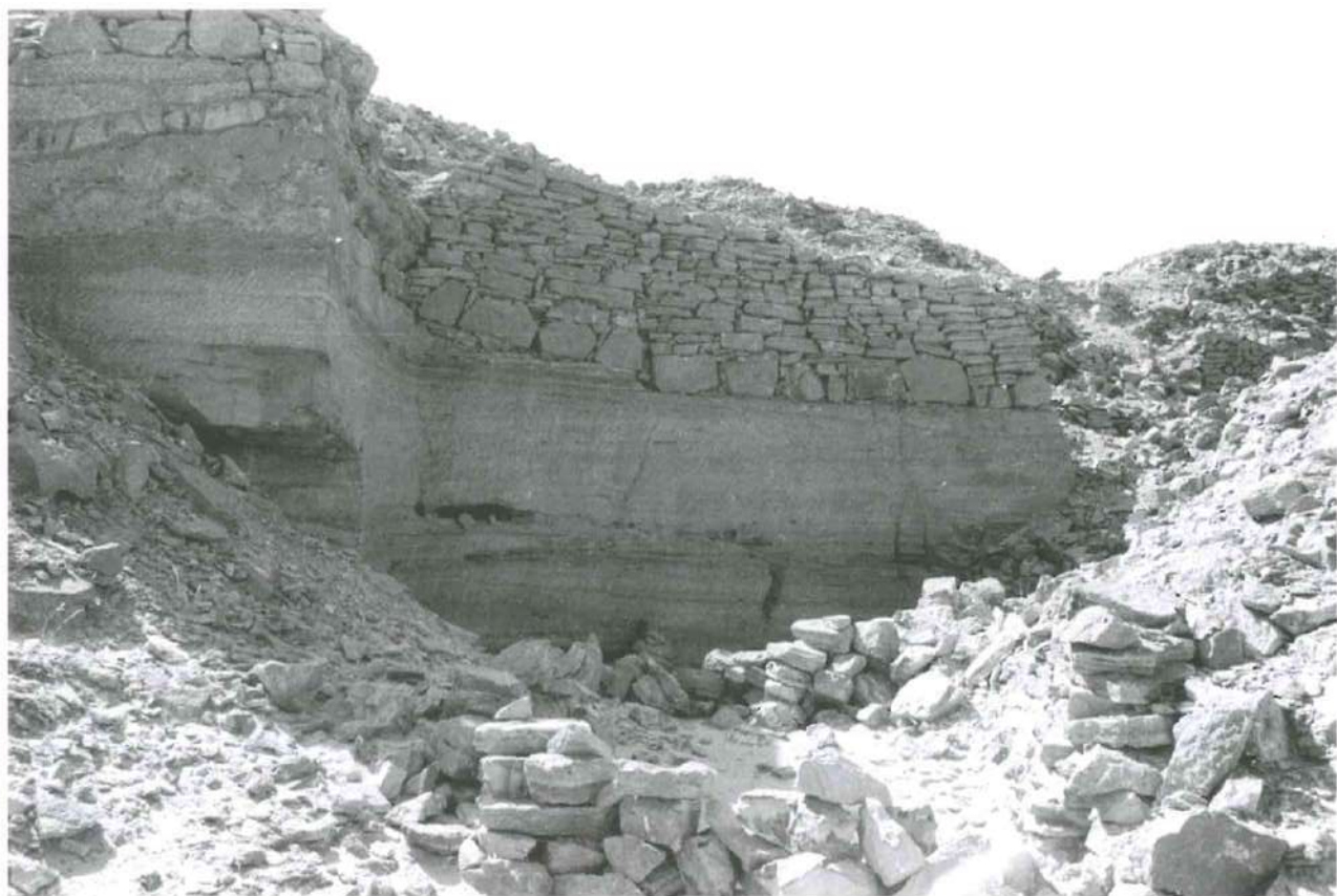
b. Al-Manqaz Quarry. A retainment wall for the excavation debris was built on the edge of the quarry.
