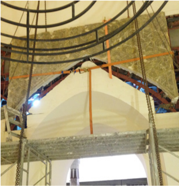
Iraq Museum repositioning of a brickwork panel on the musalla's counter-facade
