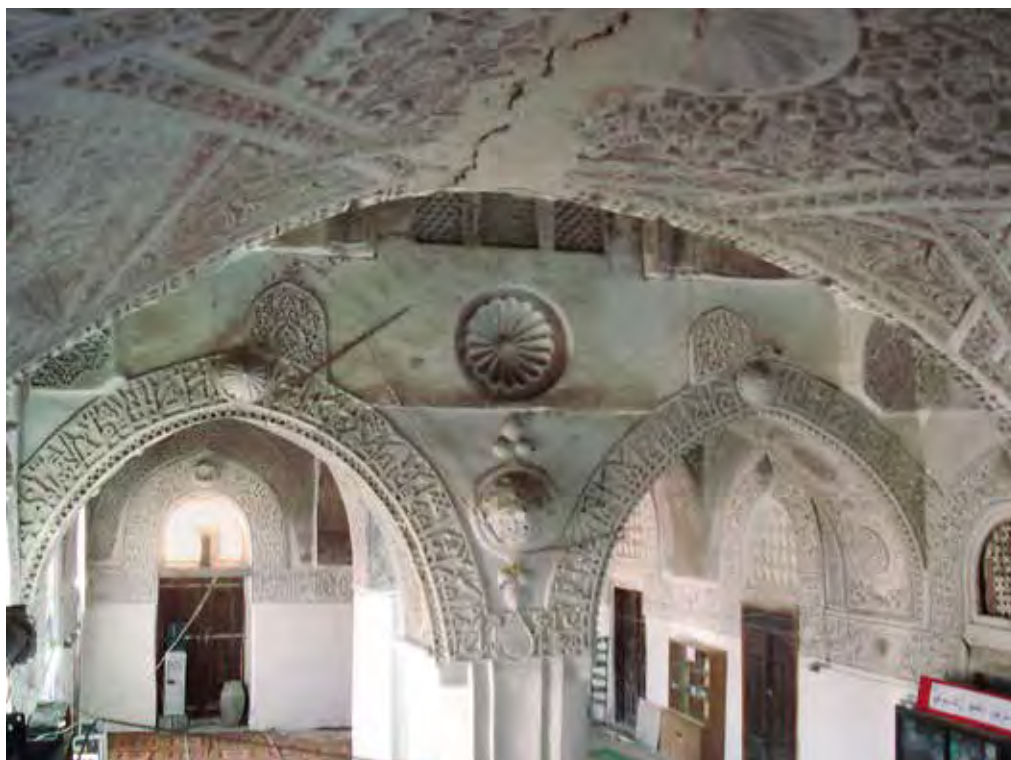
Fig. 1. Small domes. Fracture across the apex of the northwest archway.
