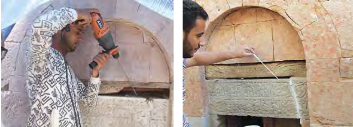
Figs. 47 and 48. Work of consolidation of the lintel, with insertion of fiberglass bars across it.
