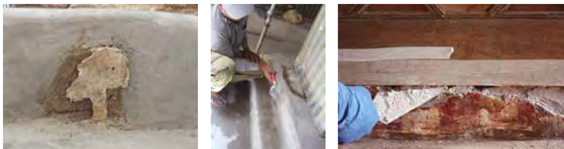
Figs. 141, 142 and 143. Views of the base of the cenotaph after removal of the plasterworks.
