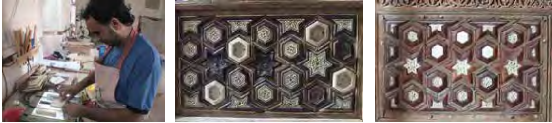
Figs. 45, 46 and 47. Stages in the work of reconstruction of the hexagonal and star-shaped inserts.
