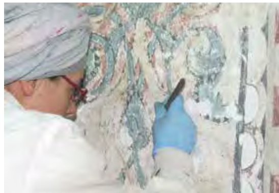
Figs. 40 and 41. Decorative band in the second register, at the height of the mihrāb . Removal of whitewash using a scalpel.
