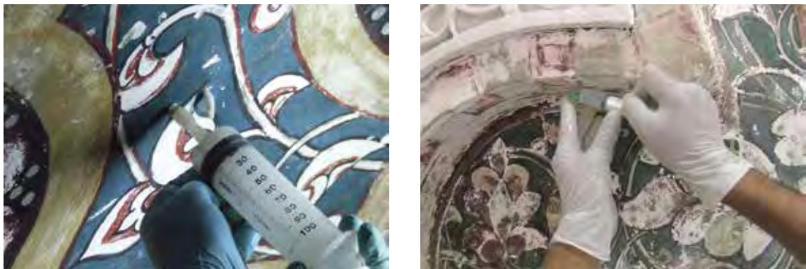
Figs. 53 and 54. Interior of dome, consolidation of plaster and polylobate arch, fixing of paint film.
