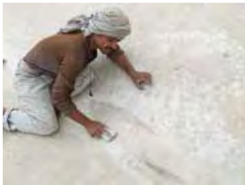
Figs. 3, 4 and 5. Workers from the building restoration company repairing cracks in the extradoses of the small domes.
