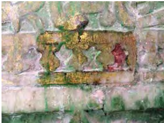
Figs. 20 and 21. Preliminary cleaning trials. Note how the gold leaf gilding of the letters is outlined by a brown edging and the spaces filled with bright red.
