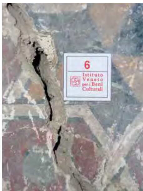
Fig. 51. Sampling point of the micro fragment of mural painting T6 with black paint taken from one of the lateral domes – al-Ashrafiyyah.
