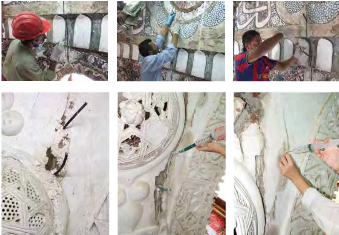
Figs. 44, 45, 46, 47, 48 and 49. Profound vertical fractures in the east and west walls. Stages in consolidation.
