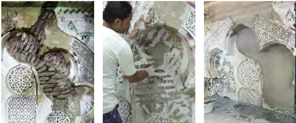
Figs. 63, 64 and 65. East wall. Polylobate arch, removal of stuccoing and stages of applying the first layer of qadāḍ plaster.
