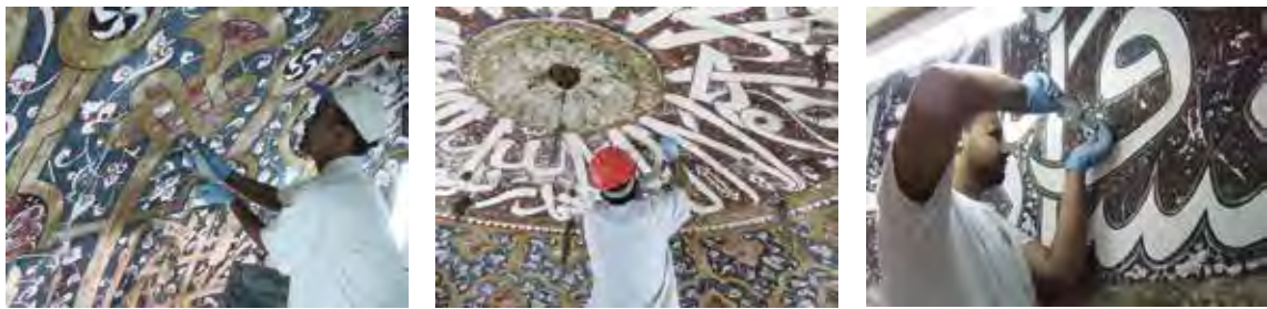
Figs. 50, 51 and 52. Interior of dome. Consolidation of detached plaster.
