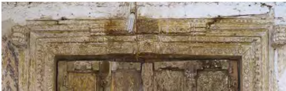
Fig. 51. Conditions of the carved lintel prior to restoration.
