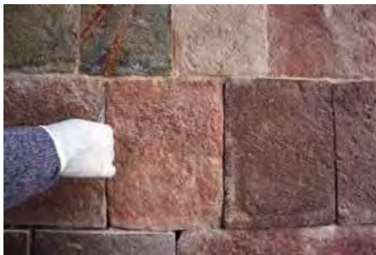
Figs. 27, 28 and 29. Stuccoing to finish the grouting between stones of the portal.
