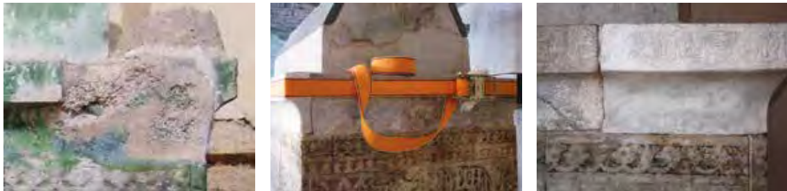
Figs. 59, 60 and 61. Views of different stages of the process of structural consolidation and insertion of a reconstructed element for completion of the Qur'anic inscription.
