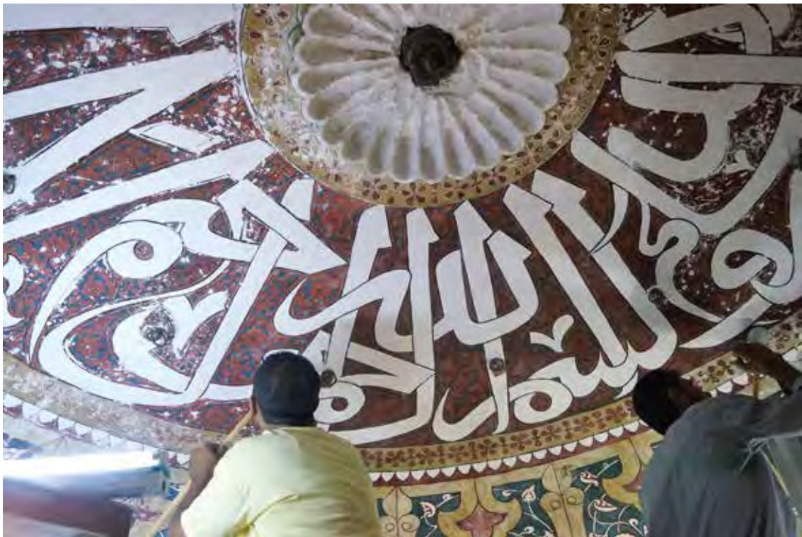
Fig. 69. Apex of the dome, the team engaged in the initial stages of retouching the basmalah in thuluth calligraphy.
