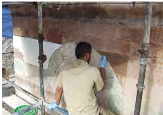
Fig. 16 and 17. Cleaning with compress of paper pulp soaked with ammonium carbonate.
