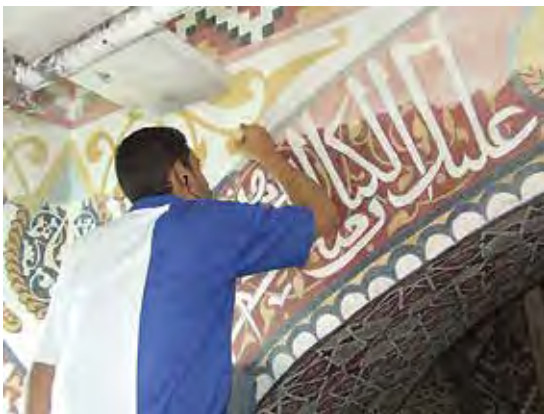
Figs. 25 and 26. Stages of restoration of painting by retouching.
