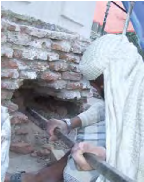
Figs. 55 and 56. Steps in replacement of beams from outside the tambour.
