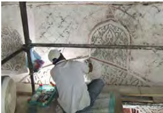
Figs. 40 and 41. Decorative band in the second register, at the height of the mihrāb . Removal of whitewash using a scalpel.
