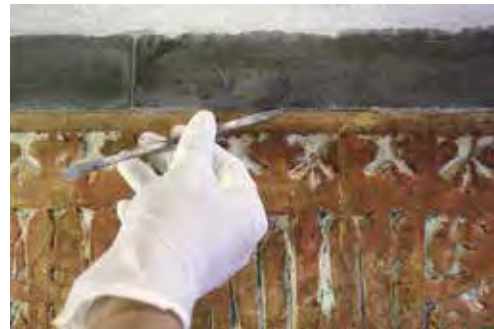
Fig. 46. Detail of the process of stuccoing the joints between the stones of the cenotaph.
