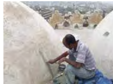
Figs. 3, 4 and 5. Workers from the building restoration company repairing cracks in the extradoses of the small domes.
