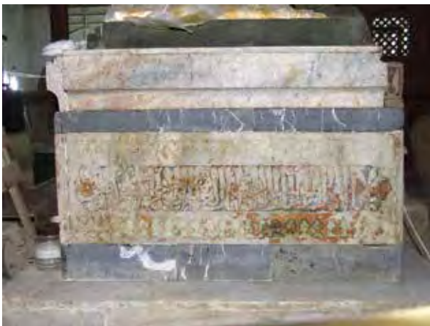
Figs. 89, 90, 91, and 92. Views of various stages of the cleaning process, including removal of old stucco patches, old disfiguring patina and the thick coating of green paint.
