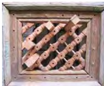
Fig. 37. Intermediate state of assembly of the reconstructed parts.
