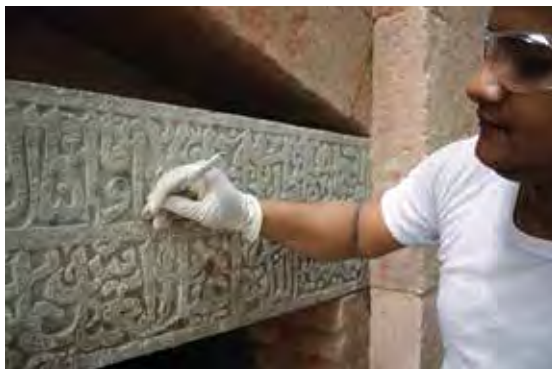
Fig. 45. Cleaning the lintel.
