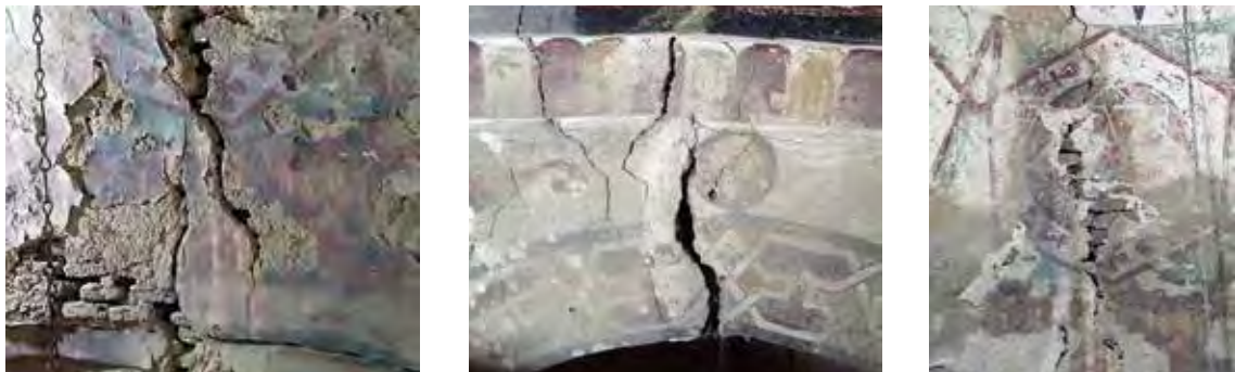
Figs. 3, 4 and 5. Small domes, fissures caused by structural sagging and detachment of the decorated plaster due to seepage.
