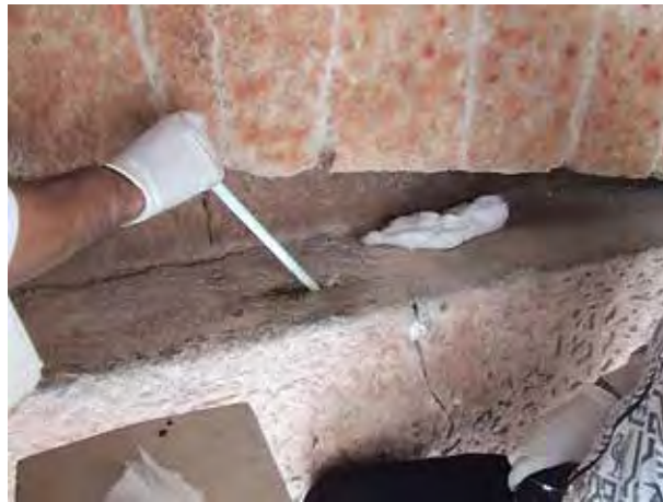
Figs. 24 and 25. Consolidation of the fractured lintel with insertion across it of bars in fiberglass.
