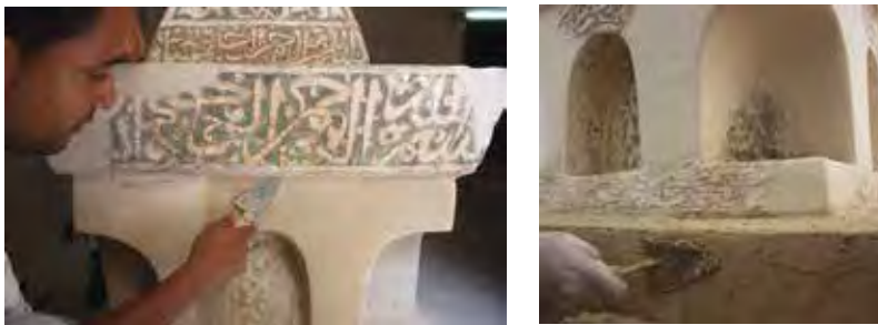
Figs. 125 and 126. Views of different stages of stucco repairs.
