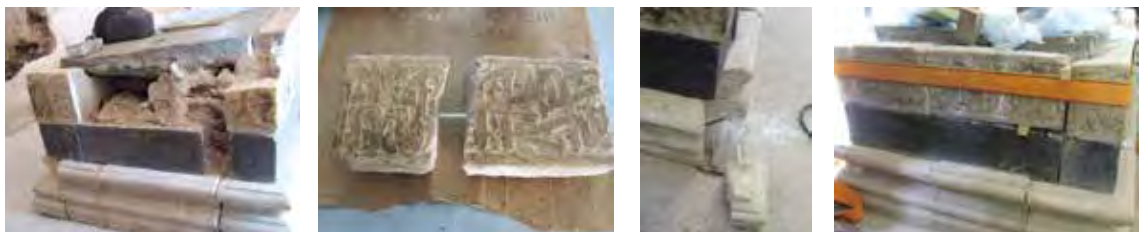
Figs. 78, 79, 80 and 81. View of different stages of the process of structural consolidation which required, among the various works, insertion of fiberglass bars.
