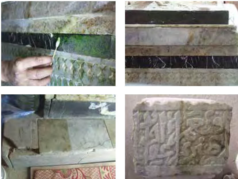
Figs. 89, 90, 91, and 92. Views of various stages of the cleaning process, including removal of old stucco patches, old disfiguring patina and the thick coating of green paint.
