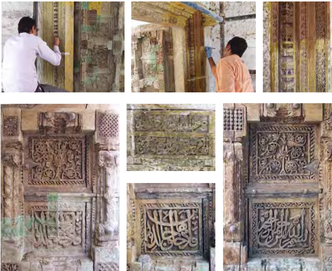
Figs. 54 to 60. Stages in the work of cleaning the doorway.
