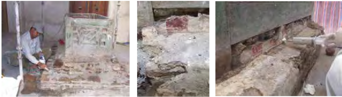
Figs. 135, 136 and 137. Views of various stages of consolidation and cleaning of the base of the cenotaph.
