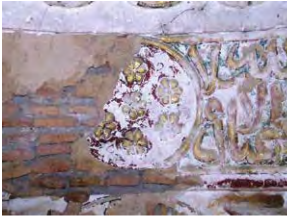
Fig. 17. Example of the effect of washout on the color of the Qur'anic inscription in dome 2a. There are also a number of white spots caused by saline incrustations scattered over the entire surface.
