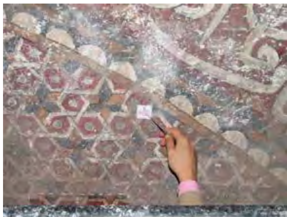
Fig. 1. Sampling point of the fragment of plaster T1 taken from lateral dome 1d - south side, under the concrete band - al-Ashrafiyyah.
