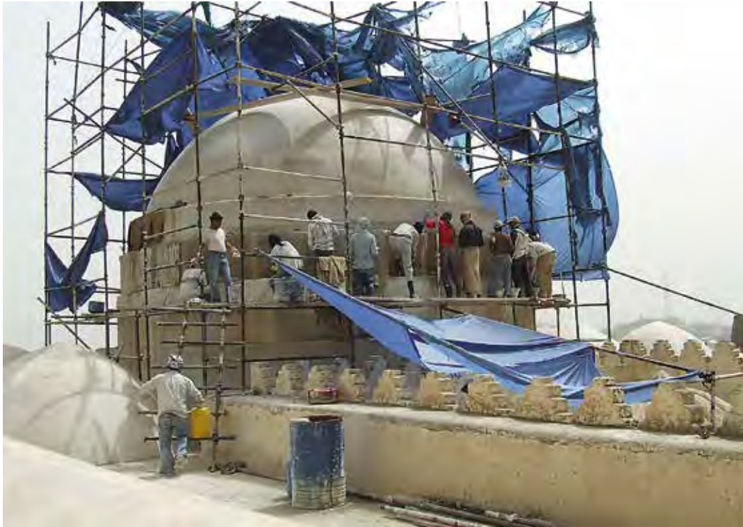
Fig. 6. The building restoration company resurfacing the qadād on the extrados of the main dome.
