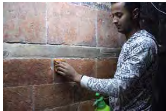
Figs. 27, 28 and 29. Stuccoing to finish the grouting between stones of the portal.
