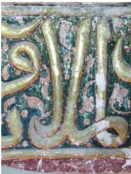
Fig. 23. Sample section of cleaning on gold Qur'anic inscription of the lower band of dome 2a.
