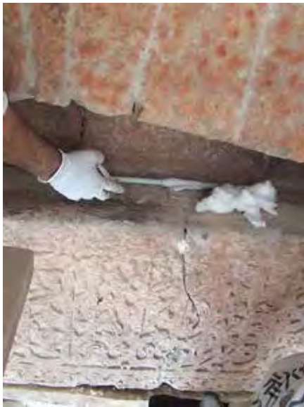
Figs. 24 and 25. Consolidation of the fractured lintel with insertion across it of bars in fiberglass.
