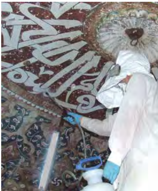
Figs. 42 and 43. Interior of dome. Stages in fixing the paint film.
