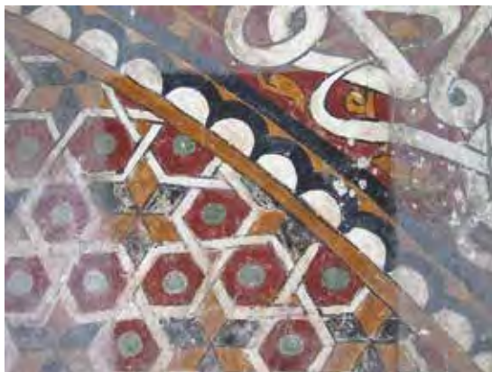
Fig. 16. West dome 1a. Cleaning test.
