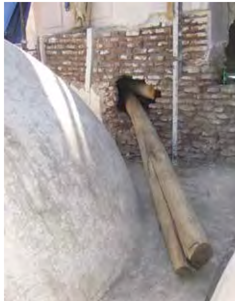
Figs. 55 and 56. Steps in replacement of beams from outside the tambour.
