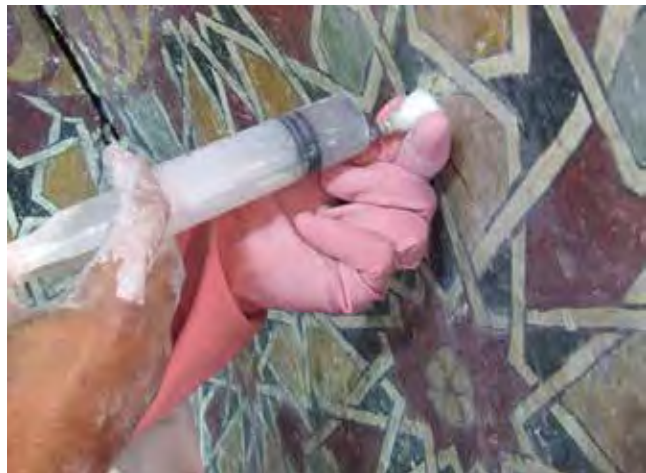
Figs. 12 and 13. Consolidation of plaster detached from a portion of the masonry.
