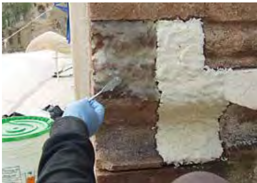
Fig. 16 and 17. Cleaning with compress of paper pulp soaked with ammonium carbonate.
