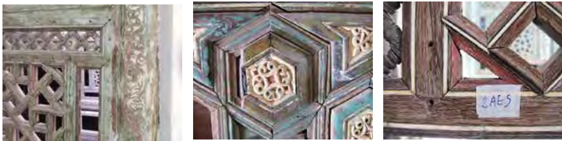
Figs. 5, 6 and 7. A few test sections cleaned to determine the state of any original painted strata.
