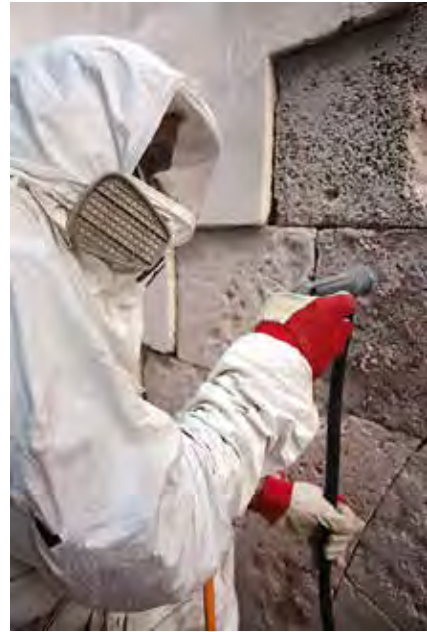
Figs. 42, 43 and 44. Cleaning the stonework portions of the portal.
