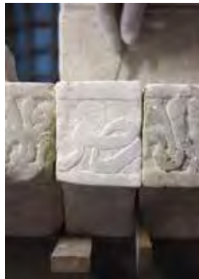
Figs. 44 and 45. Views of insertion of a reconstructed portion of the Qur'anic inscription.
