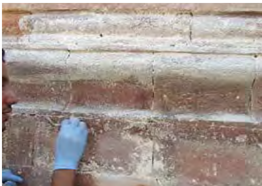
Fig. 18. Cleaning step using ion exchange resins.
