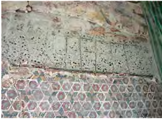
Figs. 14 and 15. Reducing the surface of the reinforced concrete beams using hammer and chisel.
