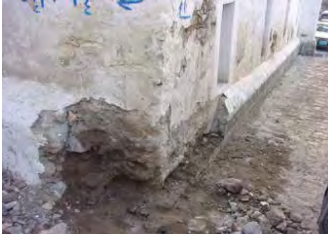
Fig. 12. Repair of the plinth at the north-eastern corner of the main building.
