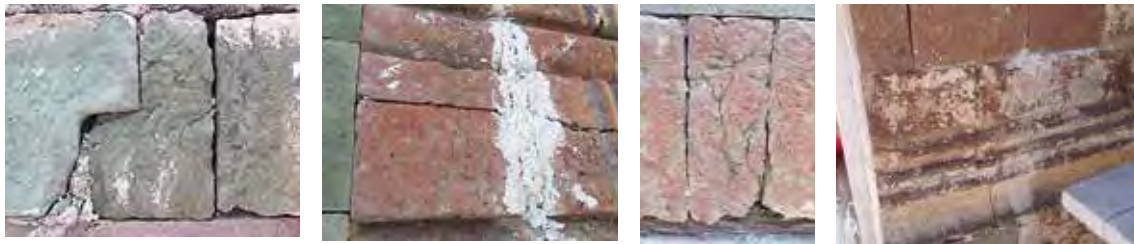
Figs. 10, 11, 12 and 13. These photos show some examples of badly done past repairs, where inappropriate techniques and unsuitable materials were used.
