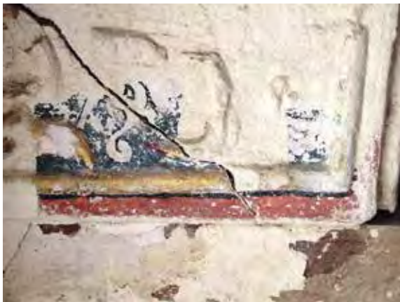
Fig. 18. Tests for removal of whitewash from the decorations of the arch in sector 2a.
