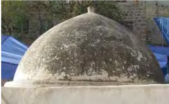
Fig. 30. Detail of the lichen covering the outside of the dome prior to starting the works.
