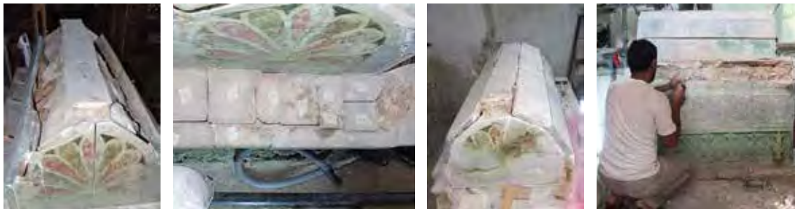
Figs. 55, 56, 57 and 58. Views of different stages of the process of structural consolidation of the cenotaph, which involved disassembly followed by complete documentation of part of its elements.
