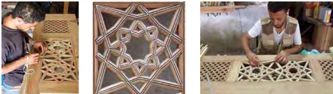
Figs. 42, 43 and 44. Stages in the work of reconstruction of the ornate geometric design of the doors.
