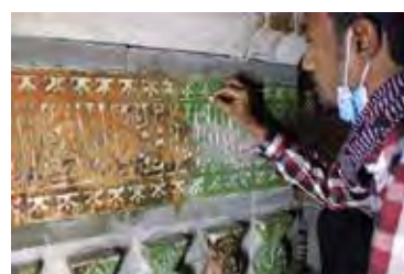
Figs. 37, 38, 39 and 40. Views of the early stages of cleaning of the gold leaf decorations on the cenotaph. The first step was solely concerned with removal of the green paint.
