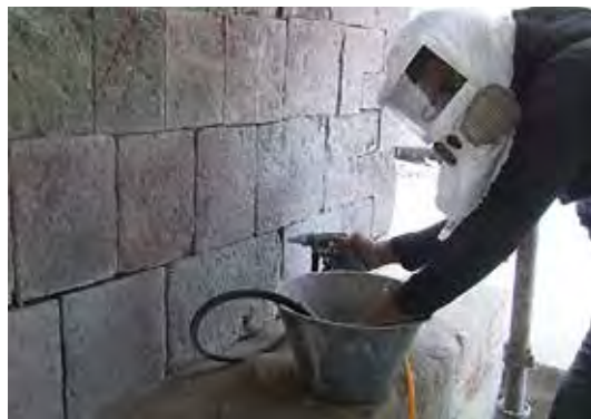
Fig. 19. Cleaning step using micro-sandblasting.
