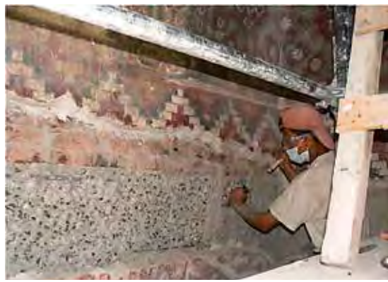
Figs. 14 and 15. Reducing the surface of the reinforced concrete beams using hammer and chisel.
