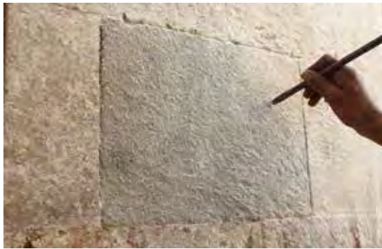
Figs. 42, 43 and 44. Cleaning the stonework portions of the portal.
