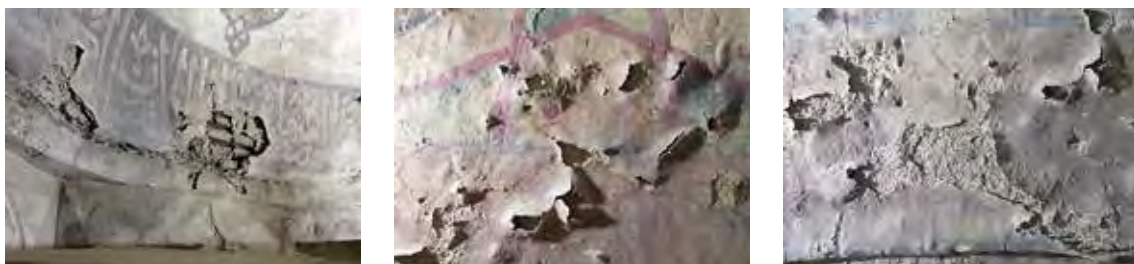
Figs. 6, 7 and 8. Small domes: examples of gaps, swelling, lifting, bubbles and powdering. Details.
