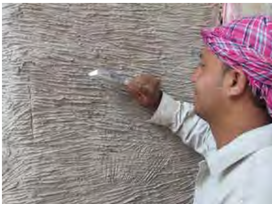
Figs. 27, 28 and 29. Example of last application with fine plaster, pounded with the sharp edge of a stone and smoothed with a flat stone during reconstruction of the qadād finish on the outer walls of al-Ashrafiyyah Mosque and Madrasah.
