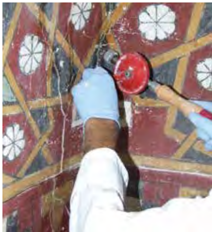
Figs. 12 and 13. Consolidation of plaster detached from a portion of the masonry.
