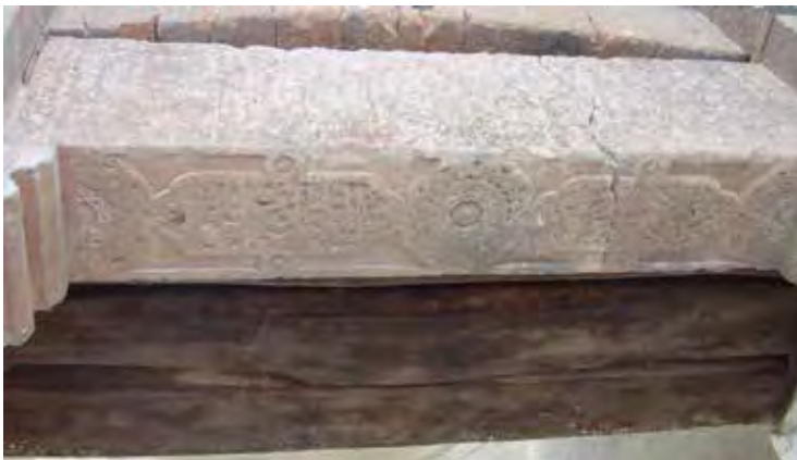
Fig. 15. Detail of the lintel with its deep fracture on the right.
