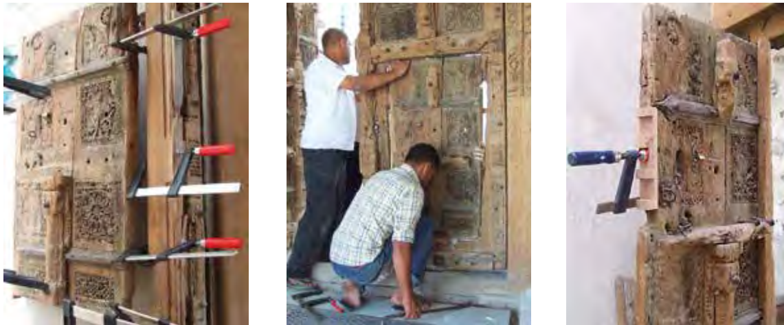
Figs. 61, 62 and 63. Stages in repairing the static conditions of the small service door in the right door panel.
