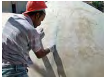
Figs. 3, 4 and 5. Workers from the building restoration company repairing cracks in the extradoses of the small domes.
