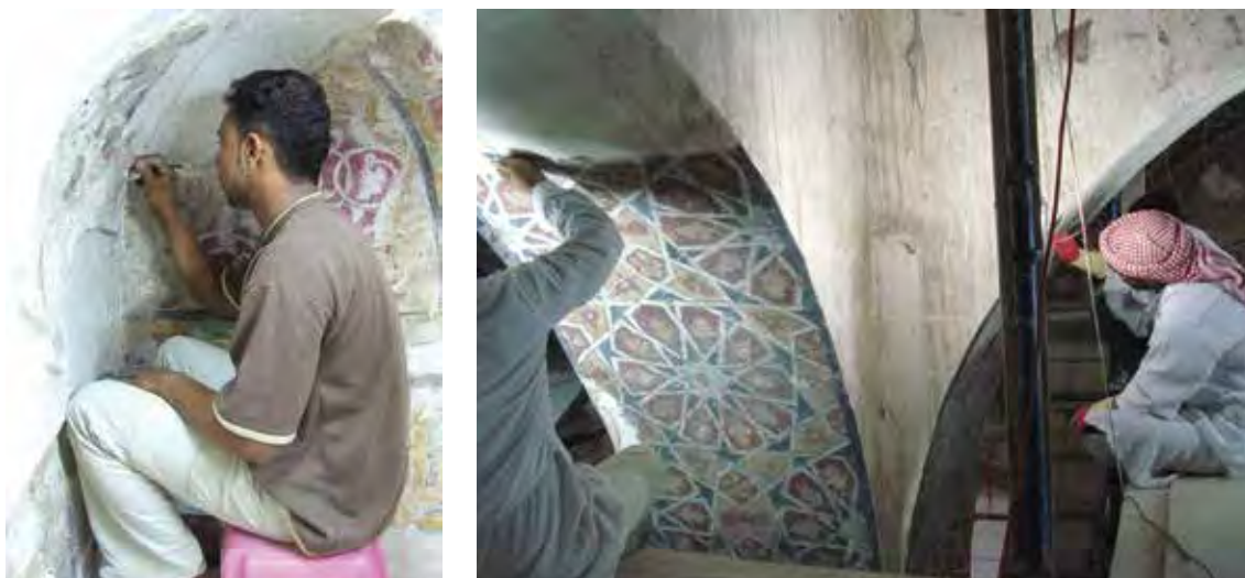
Figs. 6 and 7. Removal of lime whitewash and surface concretions using scalpels.
