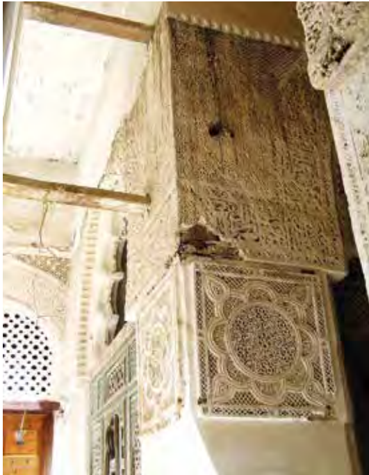
Fig. 5. Exterior stuccowork in sector 2 prior to restoration works. The geometrical design was disturbed by the thick layer of whitewash.
