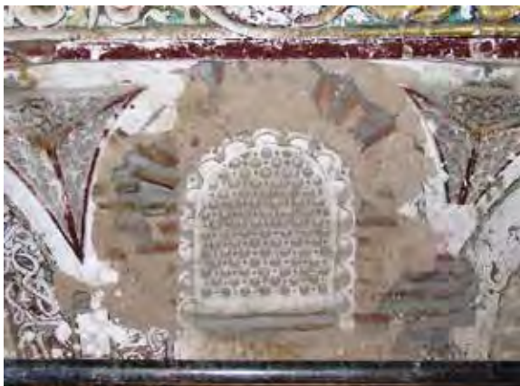
Fig. 2. Below the large gap around the window, it is possible to see the bedding mortar.
