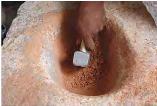
Fig. 26. Preparation of the stone powder and crushed brick that will be used to color the mortar used to grout between the stone blocks.
