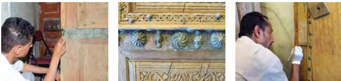
Figs. 81, 82 and 83. Steps in the cleaning of decorative elements in brass.
