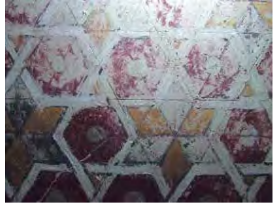
Figs. 35 and 36. Small domes: detail of repeated design made using paint-soaked cord and finished by etching.
