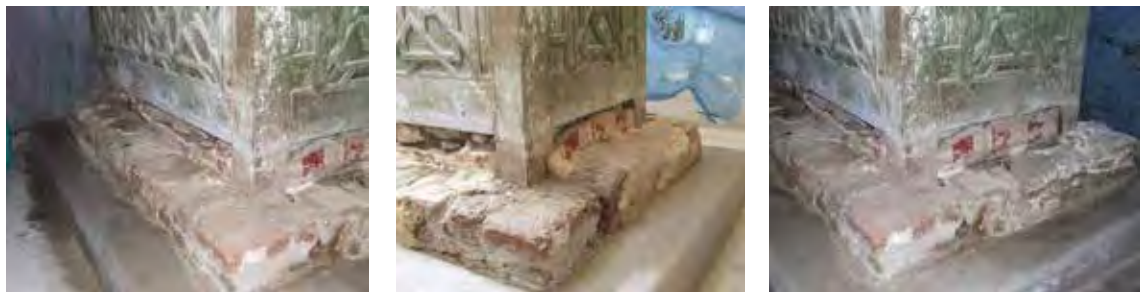
Figs. 138, 139 and 140. Views of the base of the cenotaph after removal of the plasterworks.
