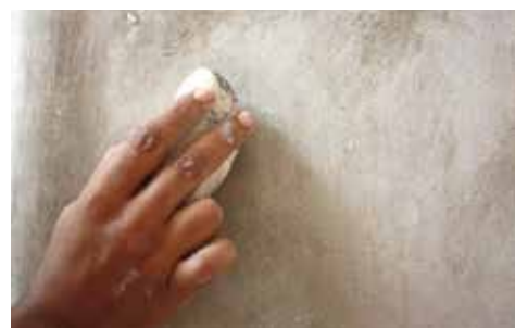
Figs. 27, 28 and 29. Example of last application with fine plaster, pounded with the sharp edge of a stone and smoothed with a flat stone during reconstruction of the qadād finish on the outer walls of al-Ashrafiyyah Mosque and Madrasah.
