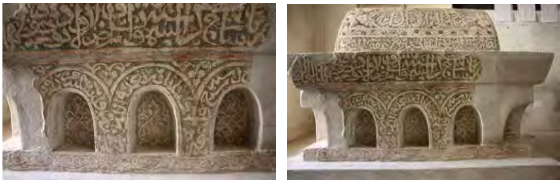
Figs. 120 and 121. Views of the cenotaph after removal of the stuccowork and with the rough plaster layer ready to receive the finishing layer of fine plaster.
