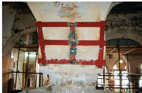
Fig. 84. Column no. 18 I, south side, cleaning and repointing of the surface.
