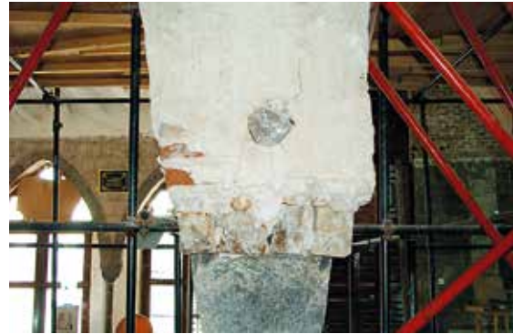
Fig. 86. Column no. 17 K, south side.
