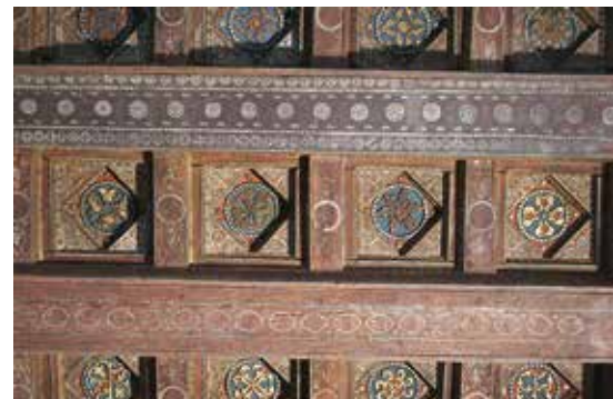
Fig. 34. Detail of the western sector at the end of the intervention.
