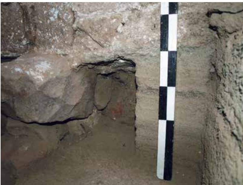
Fig. 22. Detail of the horizontal probe below the present northwest corner of the east minaret. The large stone on the left side of the photograph corresponds to the stone visible on the right side of Fig. 16. The plaster visible below this stone is the west side of the recessed shelf. Behind the scale is visible the stack of floors upon which the northwest corner of the enlarged minaret sits.
