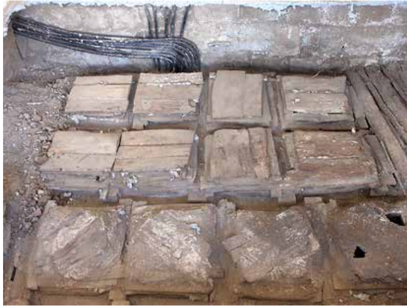
Fig. 6. The coffer free from covering material.
