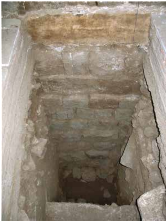
Fig. 11. Interior face of the east wall near the northeast corner of the Mosque. The wider course of stones at the bottom of the foundation may belong to an earlier structure. The wall plaster is the original plaster of the east riwāq and its bottom corresponds to the initial floor of the east riwāq .
