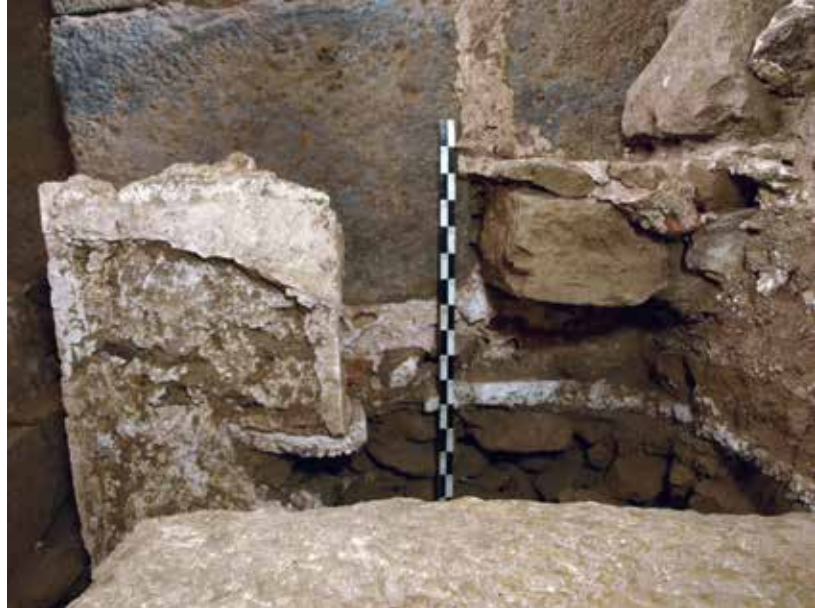
Fig. 7. Bottom of the surround at the imam's doorway, with the plastered remains of the earlier entry in front. The bottom of the surround sits upon an accumulation of plaster floors and stone rubble of the earlier entryway, but the surround has no foundations proper to it.
