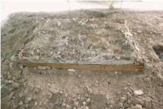
Fig. 17. Removal of the roof covering.
