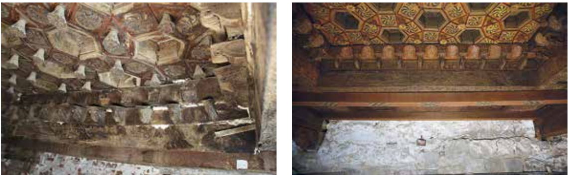
Figs 28 and 29. A comparison photos before and after restoration.
