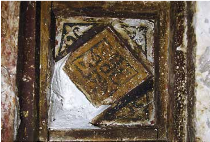
Fig. 22. Example of an old maintenance intervention that fills the lack of one of the four triangles with one plaster grouting.
