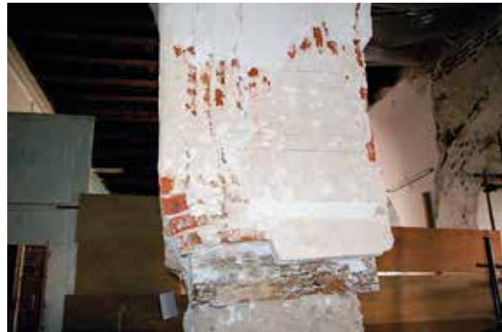
Fig. 82. Column no. 18 I, east side, cleaning and repointing of the surface.
