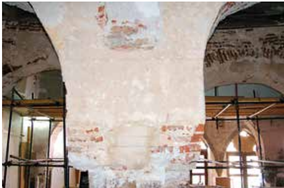
Fig. 81. Column no. 18 I, south side, cleaning and repointing of the surface.
