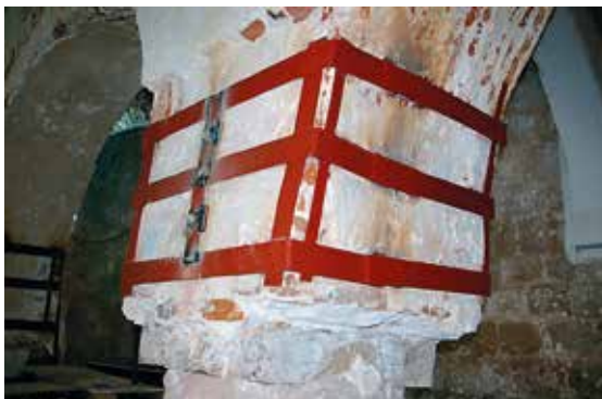
Fig. 83. Column no. 18 I, northwest side, application of metal cage.
