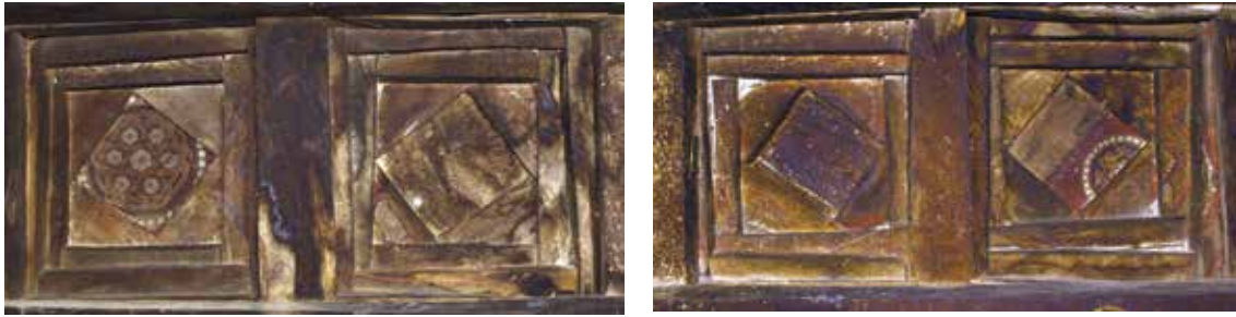
Figs 8 and 9. Some coffers in the southern sector.
