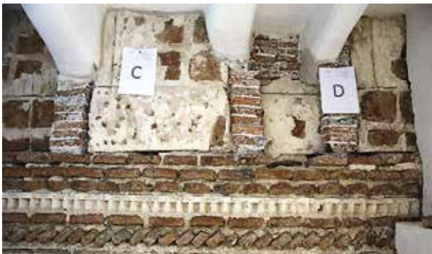
Figs 48, 49. Southeastern minaret, detail of the interior decoration before and after restoration.
