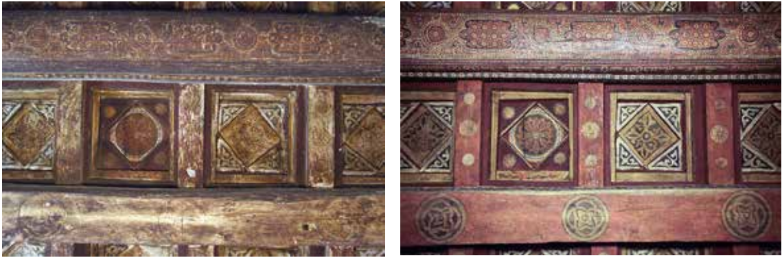
Figs 27 and 28. Detail of a portion of coffered ceiling, before and after the restoration. North sector.
