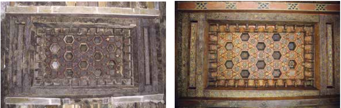
Figs 32 and 33. A comparison photos before and after restoration.
