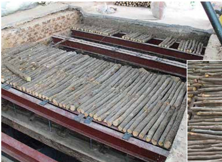
Fig. 14. First phase of closing the ceiling.
