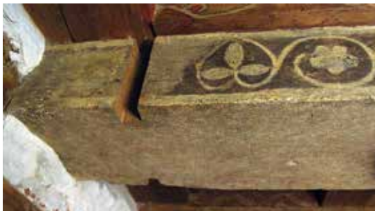
Figs 10, 11 and 12. Some examples of old exposed joints that are no longer used, reflecting a reuse of the beams.
