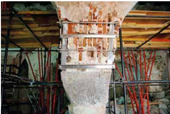
Fig. 77. Column no. 16 K north side.
