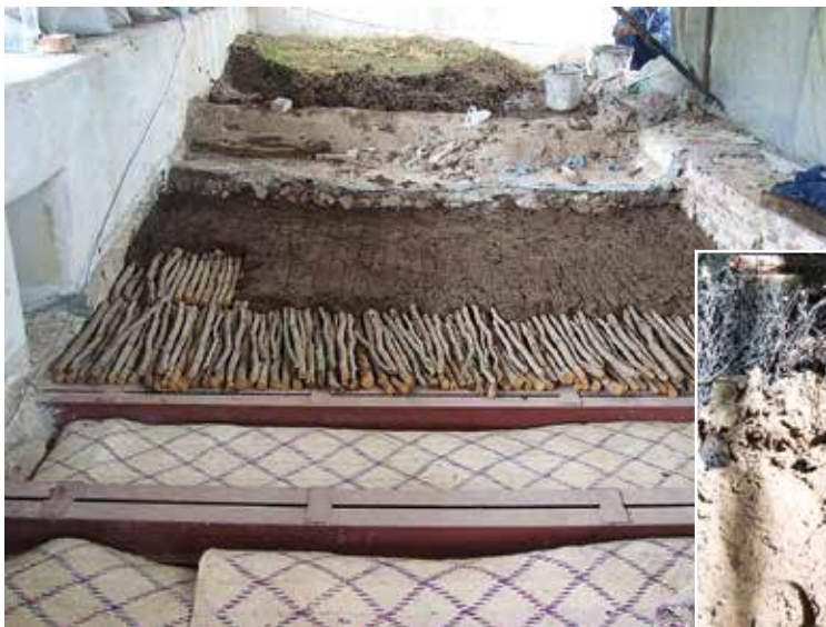
Fig. 15. Intermediate phase of closing the ceiling.
