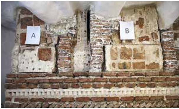
Figs 46, 47. Southeastern minaret, detail of the interior decoration before and after restoration.
