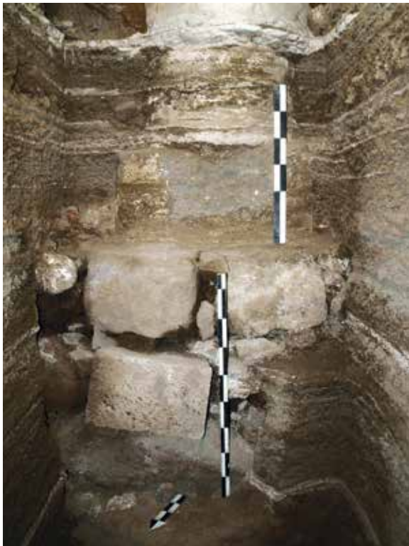
Fig. 39. Upper portion of the foundation piling, the base and pier at pillar A7 in the west riwāq . Note the recycling of dressed facing stones in the piling.
